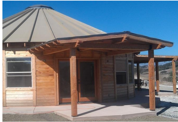
French Doors with covered entry
